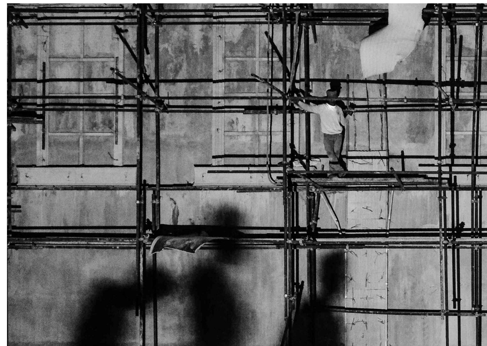
Work in Progress Aeson Baldevia
